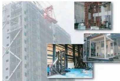
制振建築物 Seismic response control building
